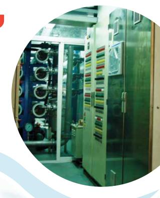
Ultrafiltration (UF) is a process of separation underpressure, Ultrafiltration (UF) is a variant of membrane-based technology. It removes a high percentage of microbes from the feed water. Its treatment process requires relatively little energy, therefore, offers a simple, chemical-free and user-friendly method of treating water.
