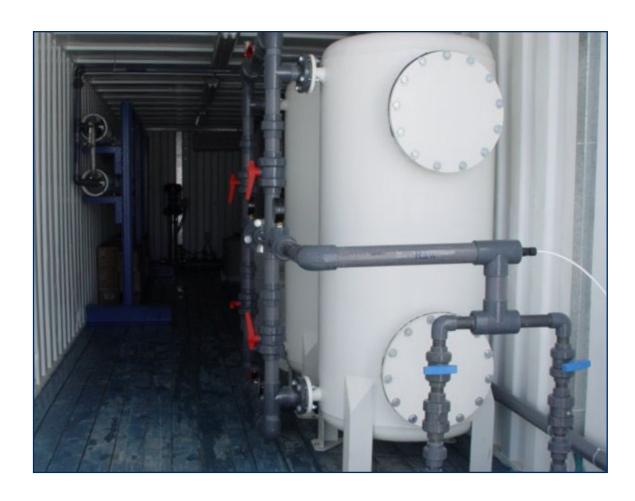
Filtration is usually used in several steps in a treatment train. Filtration captures particles of various sizes, such as clays, sands, colloids, microorganisms and organic particulates.
